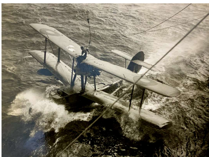
A normal recovery of Canberra's Walrus in calm seas. While Duncan manoeuvres them alongside, VAT can be seen in the right-hand seat watching the TAG attach the hook in front of the spinning propellor.
